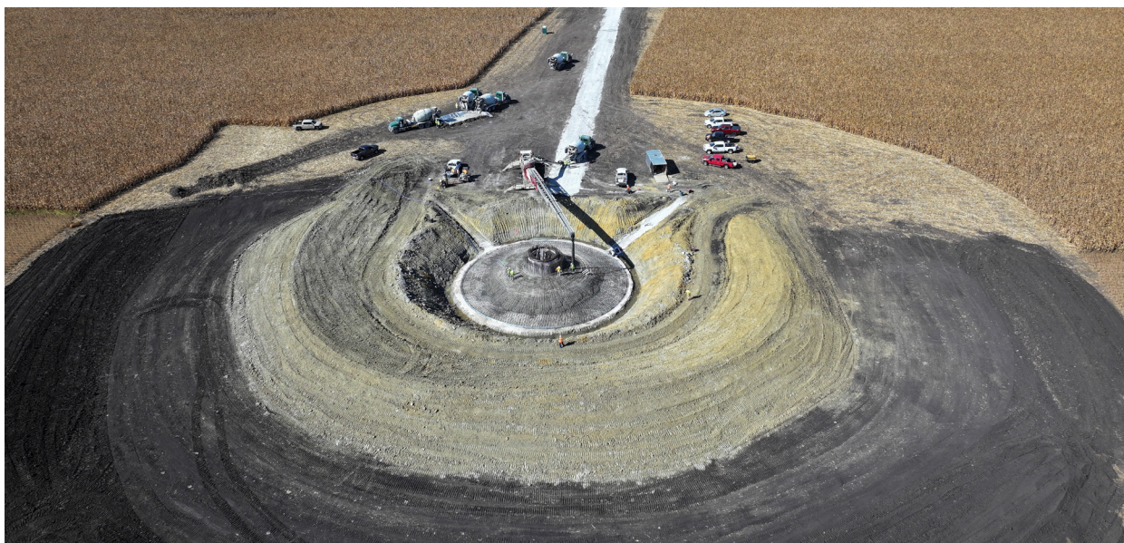
Photo: CIP, one of Panther Grove's wind turbine foundations.
